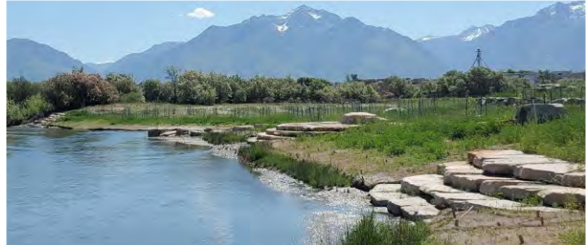
The Big Bend Project restored 70 acres of habitat for migratory birds and other wildlife by stabilizing riverbanks and constructing a new meandering channel and wetlands that will reconnect the floodplain with the river.
